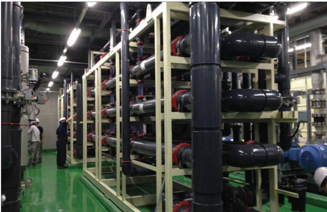
*Installed tubular membrane filtration system in operation with POREX® filter modules.*
